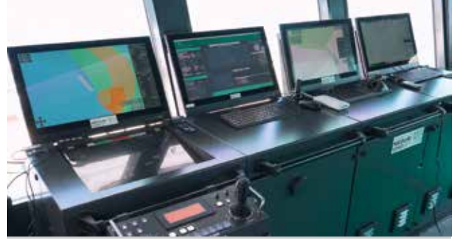
Autonomous navigation equipment installed on Olympia Dream Seto (The Nippon Foundation)
